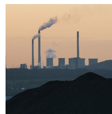
Continuous monitoring of industrial emissions
